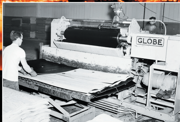
4X8 Peeled Sheets Of Wood Were Glued Together And Pressed In This Machine – Harold Keller Photo
